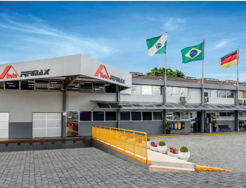
Roto Ferman headquarters in Colombo, Paraná, Brazil.
